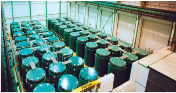
Figure 4 About 5,000 irradiated fuel assemblies are stored in this Czech interim storage facility, enough to heat up Prague for 50 years.
